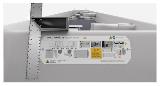
**Technique 2:** Visually, place the template in the desired installation location. Using a level, check that the template is level.
