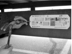
4. Remove the template. If there are any burrs around the holes, remove them. Also, remove any dust or debris left over from the drilling or de-burring operations.
