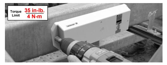
Tip: if you choose to use a self-drilling screw on an installation surface whose construction leaves the sharp point of the screw exposed, you may wish to remove the pointed end of the screw after the module is mounted to the chassis. This can prevent possible injury, or damage, from the exposed screw ends.
