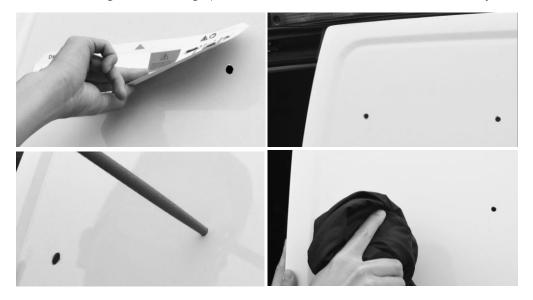
5. Remove the liner from the mounting pads, to reveal the adhesive. **IMPORTANT:** This adhesive is intended only for temporary assistance during product installation. Do not attempt long term product usage without the use of fasteners.
