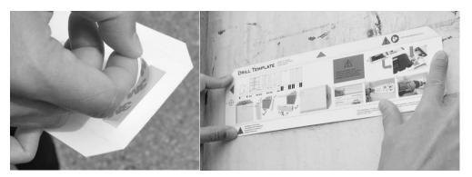
It is recommended that you install the module as level as possible on the asset. Angled installations are not supported. To help ensure the module is level, you may try one of the following techniques.
