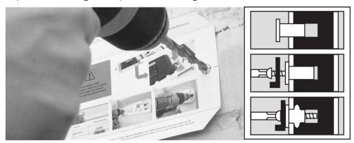
5. Remove the template. You now have two holes in the door. If there are any burrs around the holes, remove them at this time. Also, remove any dust or debris left over from the drilling or de-burring operations and ensure surface is clean and dry.
