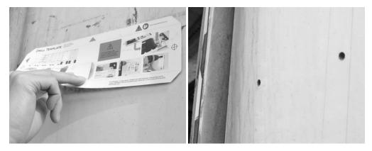
**Tip:** If you are planning to use well nuts as part of your installation, you may insert the well nuts in the holes, at this time. Skip to Step 7, as you will not need to use the mounting adhesive to install the module.
