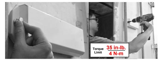
Do not over-tighten the fastener. Over-tightening can over-compress the mounting pad, which can damage the pad. Do not tighten fastener beyond 35 in-lb. (4N-m).
