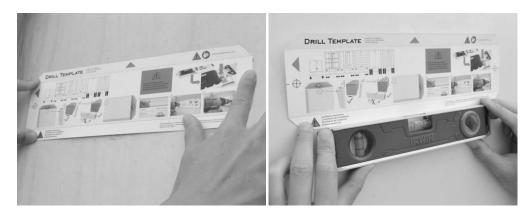
4. Using a drill bit, drill a hole through each of the cross hairs on the template. This will create two holes you will use to mount the module.
