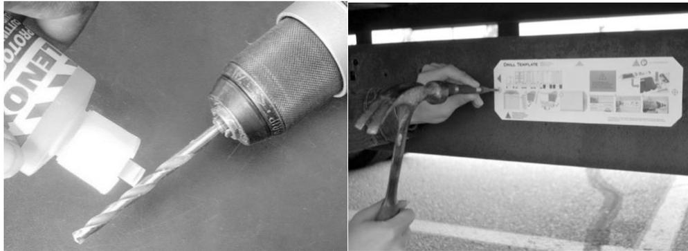
4. Remove the template. If there are any burrs around the holes, remove them. Also, remove any dust or debris left over from the drilling or de-burring operations.
