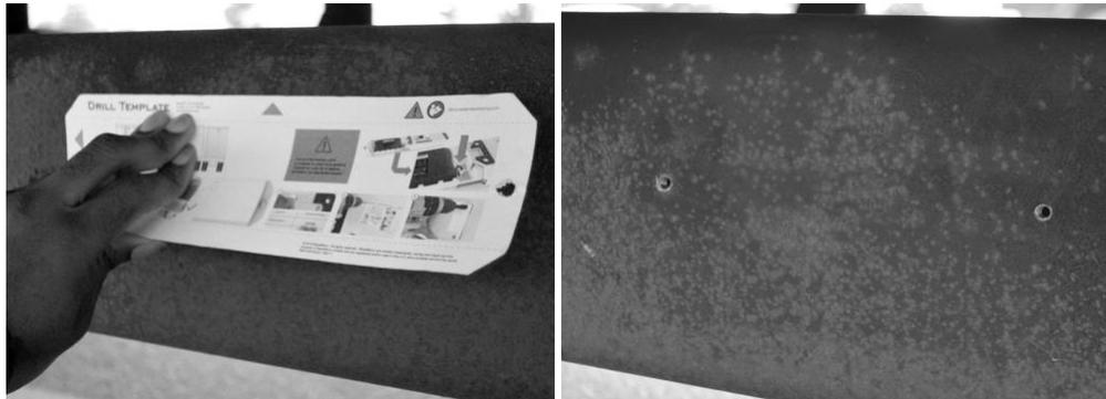
5. Place the module on the chassis, aligning the holes on the module with the holes you drilled into the asset.
