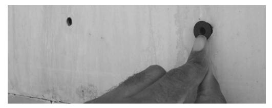
7. Mount the module to the door using one of the approaches below. The recommended procedure will differ slightly based on desired door placement and fastener selection.
