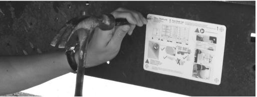
4. Remove the template. If there are any burrs around the holes, remove them. Also, remove any dust or debris left over from the drilling or de-burring operations.
