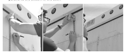
4. Remove the adhesive from the rear of the template and place the template in the desired installation location. The adhesive at the back of the template ensures that it stays on the door surface for accurate drilling of your holes.
