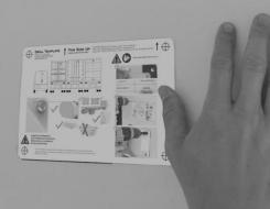
5. Using a drill bit, drill a hole through each of the cross hairs on the template. This will create four holes you will use to mount the module.
