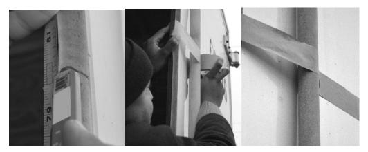
**Tip:** For trailers and containers with roll-up doors--once you have identified the desired placement height for your installation--take two measurements for location, marking each point on the exterior wall, then draw a straight line between the two points. This will ensure your line is parallel to the bottom of the door.
