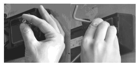
**Tip:** For faster screw installation, you may install using a 5mm hex bit on a cordless drill. If you use a drill to install the screws, please use caution to avoid over tightening (do not exceed 48 in-lb. or 5 N-m).
