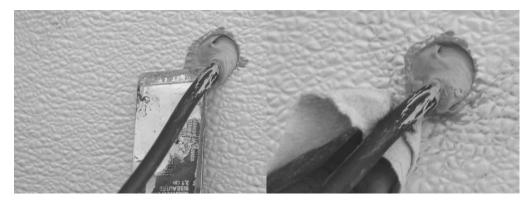
14. From inside the container, locate the cable, and guide the cable connector through the hole at the rear of the internal module. Guide internal module along the cable, towards the door.
