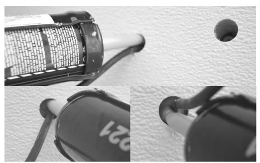
13. If the sealant expands on to the internal door surface, be sure to remove the excess insulation from the door surface. To successfully complete the installation, it is important the device is installed flush to the installation surface. Excess sealant can be removed with a putty knife, and a towel saturated with alcohol.
