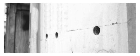
2. Source a set of plugs (nylon, rubber or metal), of the appropriate diameter, to fill the holes. These plugs can be sourced from hardware or auto supply stores. Insert the plugs into the holes. If desired, you may add 100% Silicone Exterior Grade caulk to the rear of the plug for extra protection to seal any gaps against water entry.
