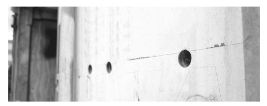
2. Source a set of elevator bolts, washers, and nuts to fill the holes. The outer surface diameter of the bolt should exceed the diameter of the hole to be covered. Insert the bolt into the hole. Place a washer between the nut and the interior door surface, and tighten the nut securely to the bolt.
