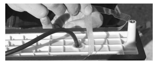
9. Locate the cable and guide the cable connector and the cable through the middle hole (Hole B on the drill template).
