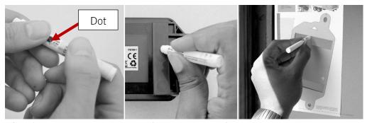
**Tip:** If you have removed the perforated sections from the Installation Template, apply the primer within the openings. These openings will precisely identify areas where the 3M VHB Universal Primer will be applied to the installation surface.
