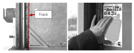
**Technique 2:** Visually, align the dotted line near the bottom of the template to the mark you created on the wall. Using a square or level, confirm that the template is level and the bottom edge of the template is parallel to the floor.
