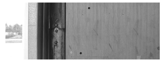
2. Fill the holes with a weatherproof sealant. If desired, you may use 100% Silicone Exterior Grade caulk or Polyurethane Sealant.
